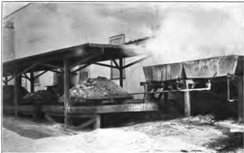
A. EVAPORATION AND CRYSTALLIZING PANS FOR RECOVERY OF SODIUM NITRATE.
